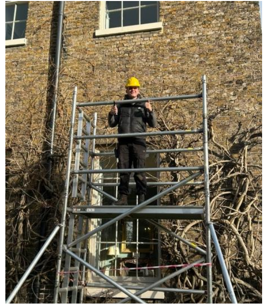
Pruning the Wisteria Senensis on the Palace wall on the scaffold structure
